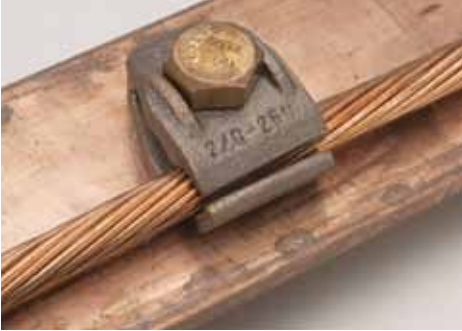
Grounding to flat surfaces
