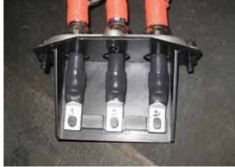
Grounding wire to steel
