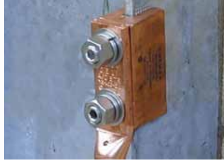
Grounding to I-beam or structural steel
