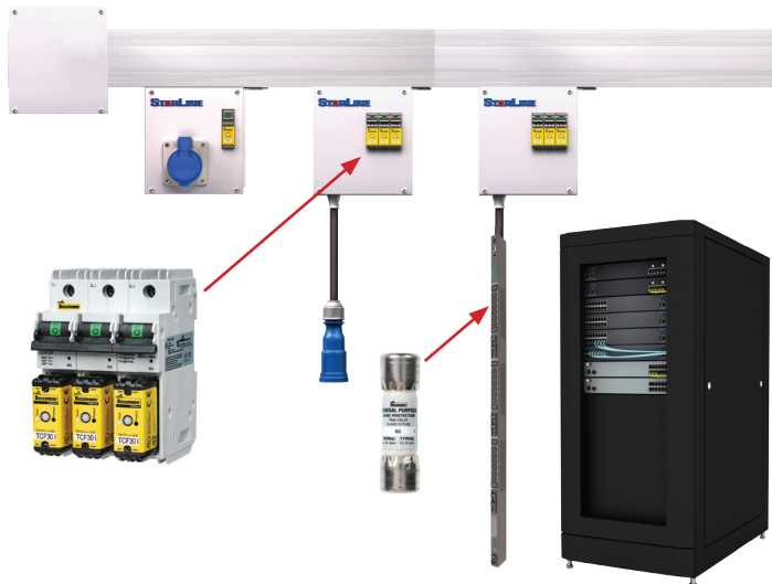
Figure 13. StarLine® Track Busway fusible disconnects utilizing CCP with CUBEFuse feeding ServerTech rack PDU utilizing the CCPLP with SC fuses.
