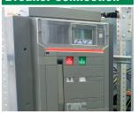
Sends trip signal to breaker trip coil (undervoltage or shunt trip) to interrupt power. Ability to trip upstream breaker if local breaker fails.
